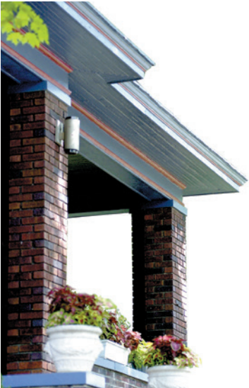
Box-gutters are wide overhanging eaves encase the gutter
