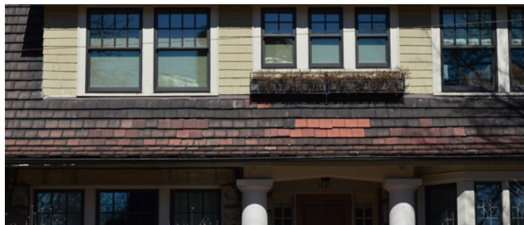
Patch and maintain the roof instead of waiting until it needs replacing.
