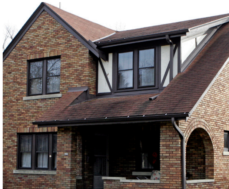
Compatible exterior storm windows should align with the window pane size and configuration.
