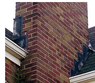
Inspect flashing for water leaks.
