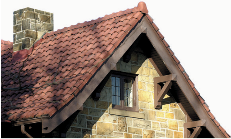
Triangular knee braces, open eaves and flared roof line
