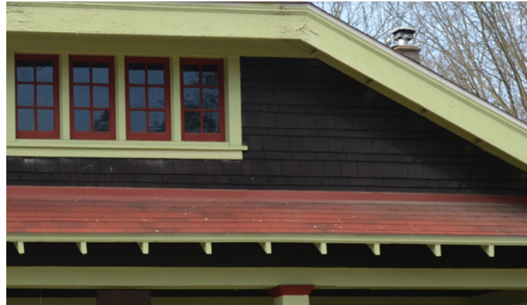
Patch and stain or paint shingles to maintain shingle quality or the home's style.
