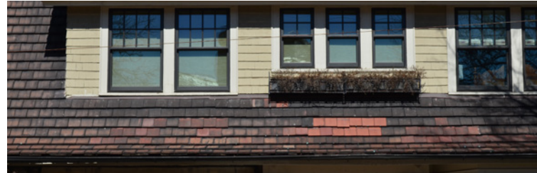
Patch and maintain roof instead of waiting until it needs replacing.
