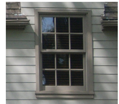
Double-hung windows are seen on Colonial Revival, Foursquare, and Craftsman houses.
