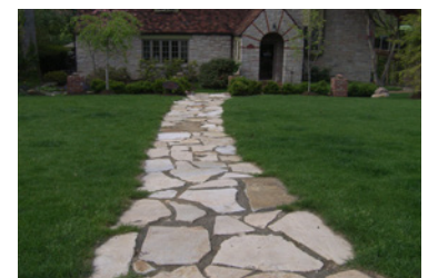
Pervious path reduces rainwater runoff
