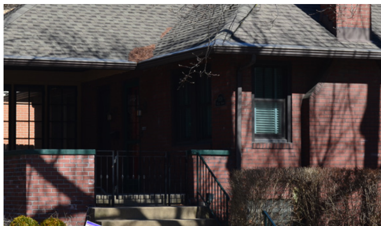
Incorrect repointing can lead to cracks and brick or mortar deterioration. This example shows a porch and chimney repointed correctly with a lighter mortar.
