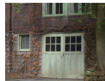
Remove moss and vines to preserve brick and stone; remove tree to maintain foundation's integrity; paint or stain wood to prevent wood decay and rot.
