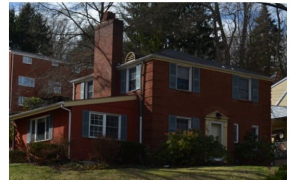
This side addition appears to be tacked-on with inconsistent materials
