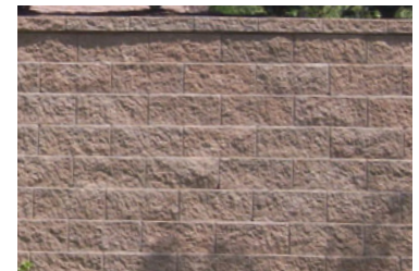
Concrete block walls inappropriate for historic homes
