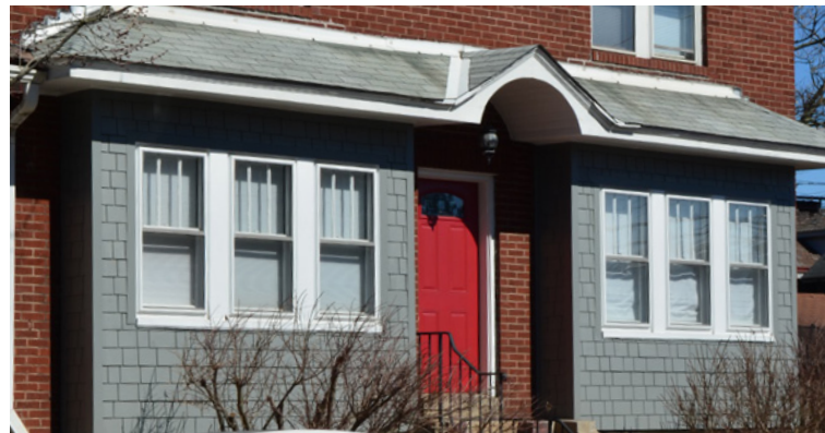
Shingle replacement matches the original shingle style (material, size, and shape).
