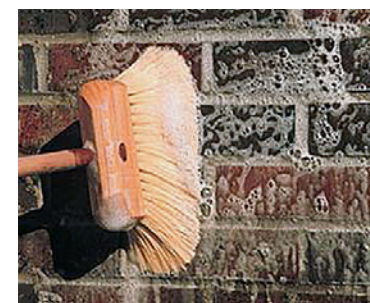
Clean brick with low-pressure water and mild detergent. Do NOT use a pressure-washer on historic brick.
