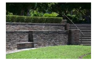
A retaining wall greater than 4 feet in height is required to have a minimum 48" high safety fence along its top where a fall hazard is present. Fences shall comply with Section 808 of Chapter XX in Mt Lebanon Zoning Ordinance.
